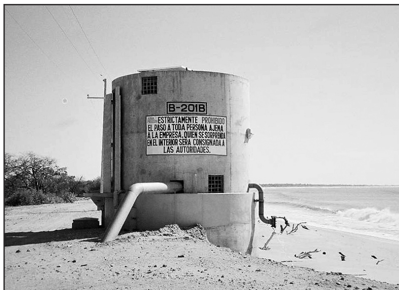
Figure 4-1 3.8 MGD intake beach well of a large seawater desalination plant
